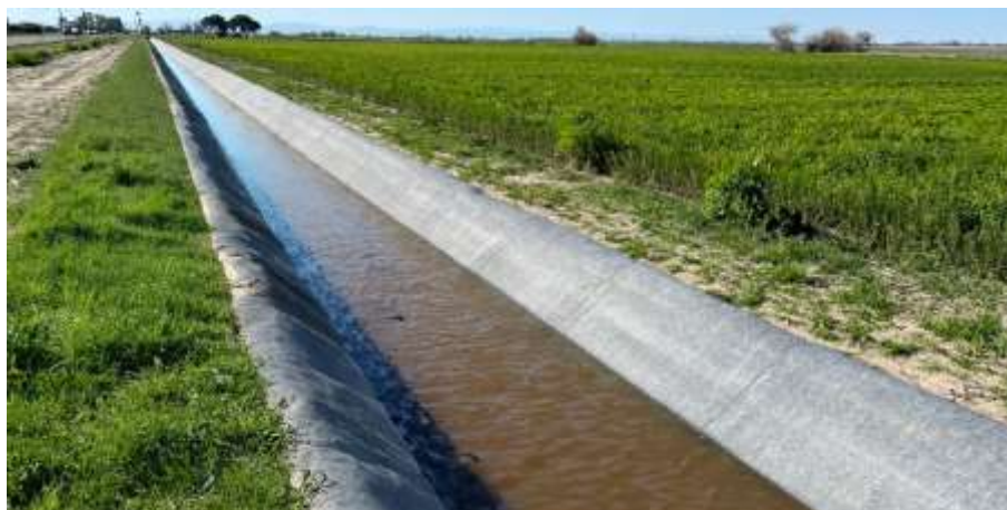
Figure 6. GCCM lined canal in operation, Henry Miller Reclamation District
