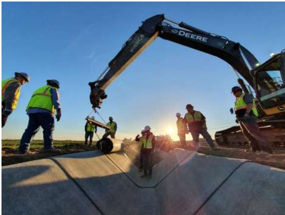
Figure 5. GCCM installation
