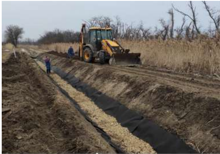
Figure 2. Installation of geotextile, gravel, and anchor trenches
